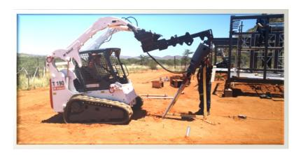
The helical anchors were all installed at an inclination angle of 60 degrees relative to the natural ground horizon and inline with the tent guy cables. The guy cables were tensioned to stretch the expanded roof tents which are supported by vertical struts along the perimeter of the expanded roof.
