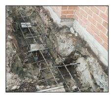
SSRG installed these piles in varying weather conditions with rain. New construction pile caps typically 8"x 8" size, used to connect the piles and new grade beam. Soil comprised of highly plastic clays overlying weathered shale and bedrock. Helical pile tip bearing on good strength shale or bedrock.
